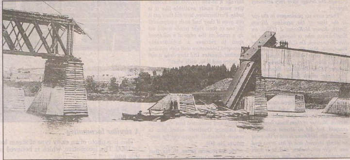
Over 100 years ago Collapse of the CPR railway bridge crossing the St. John River on June 21, 1900.
